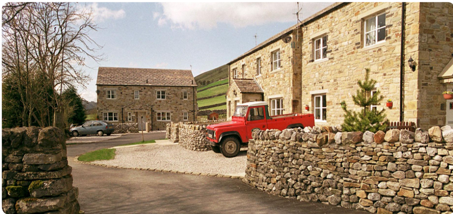
Affordable housing at Cam Garth, Craven.
